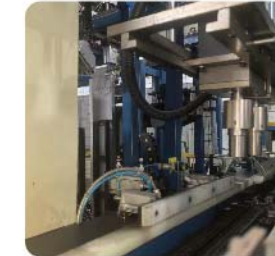
1.极柱端子矫正 1. Pole terminal correction
