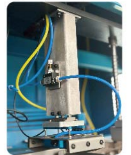
4.隔板上料 4. Plate material
